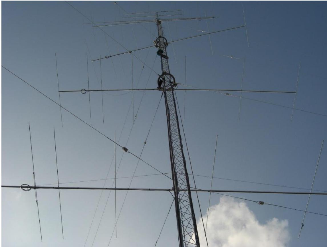
7x7x7x7 50 MHz Array at W5ZN
