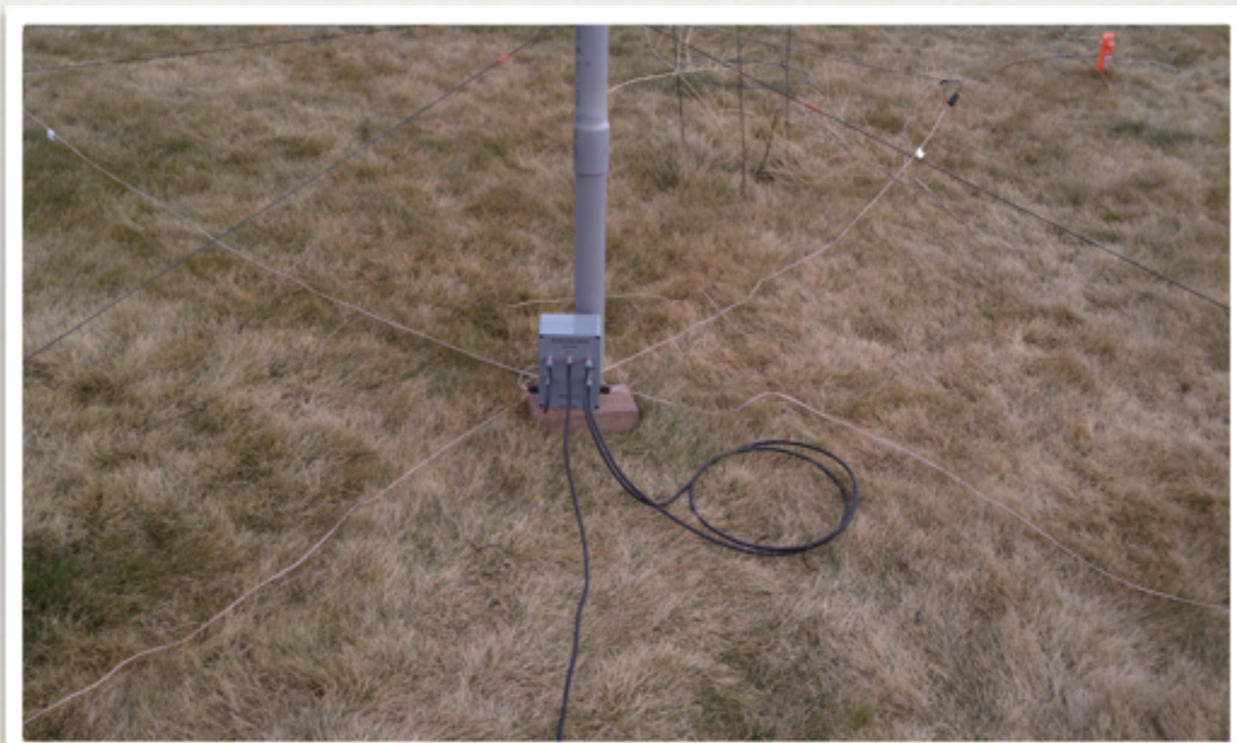
Switch Assembly at Base of Shared Apex Loop Array
