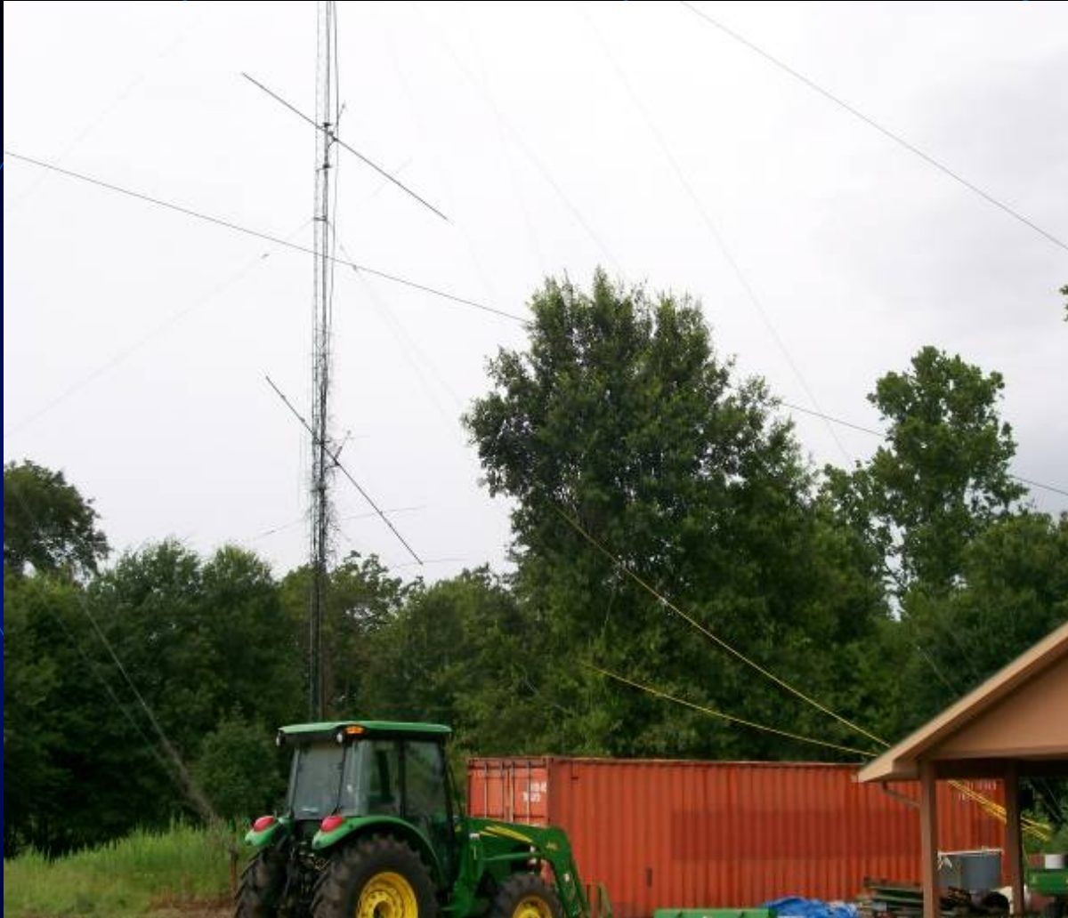
Damaged 10M stack tower
