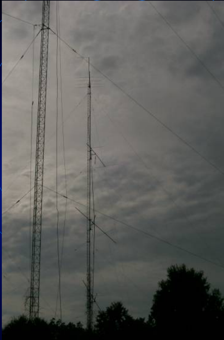
Damaged 15M stack tower
